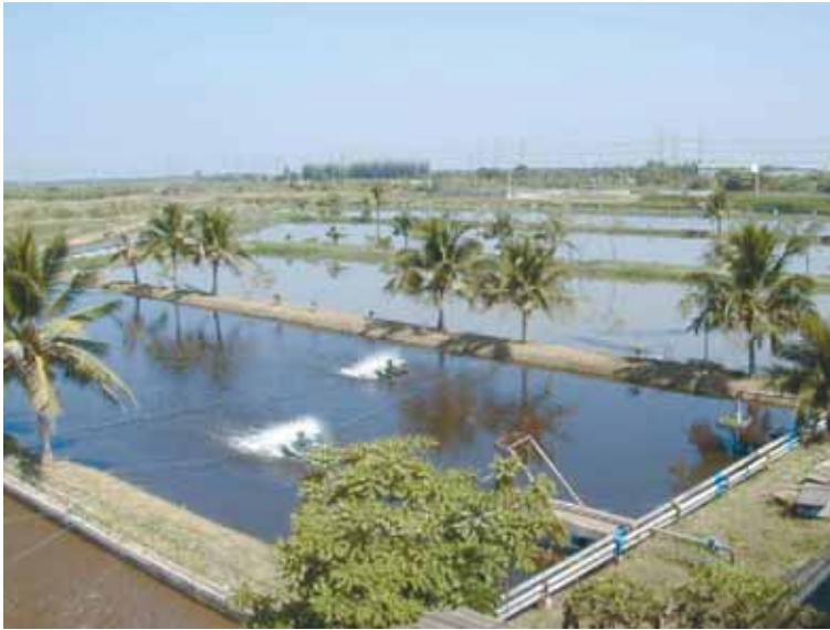
The waste-water treatment installation of a Thai chicken manufacturer, who exports meat to OECD countries.
